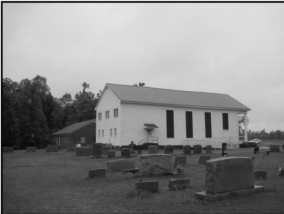
Figure 61. No. 79 Carvers Creek Methodist Church, Church and Setting, Looking North
