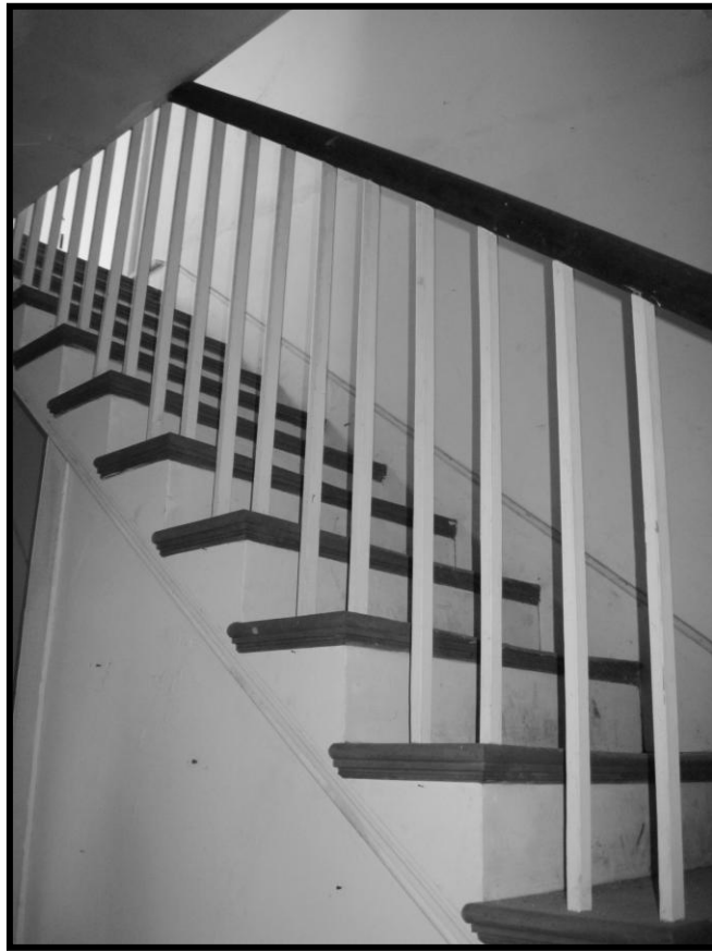
Figure 71. No. 126 Love House, Interior, First Floor, Detail of Stair, Looking East.
