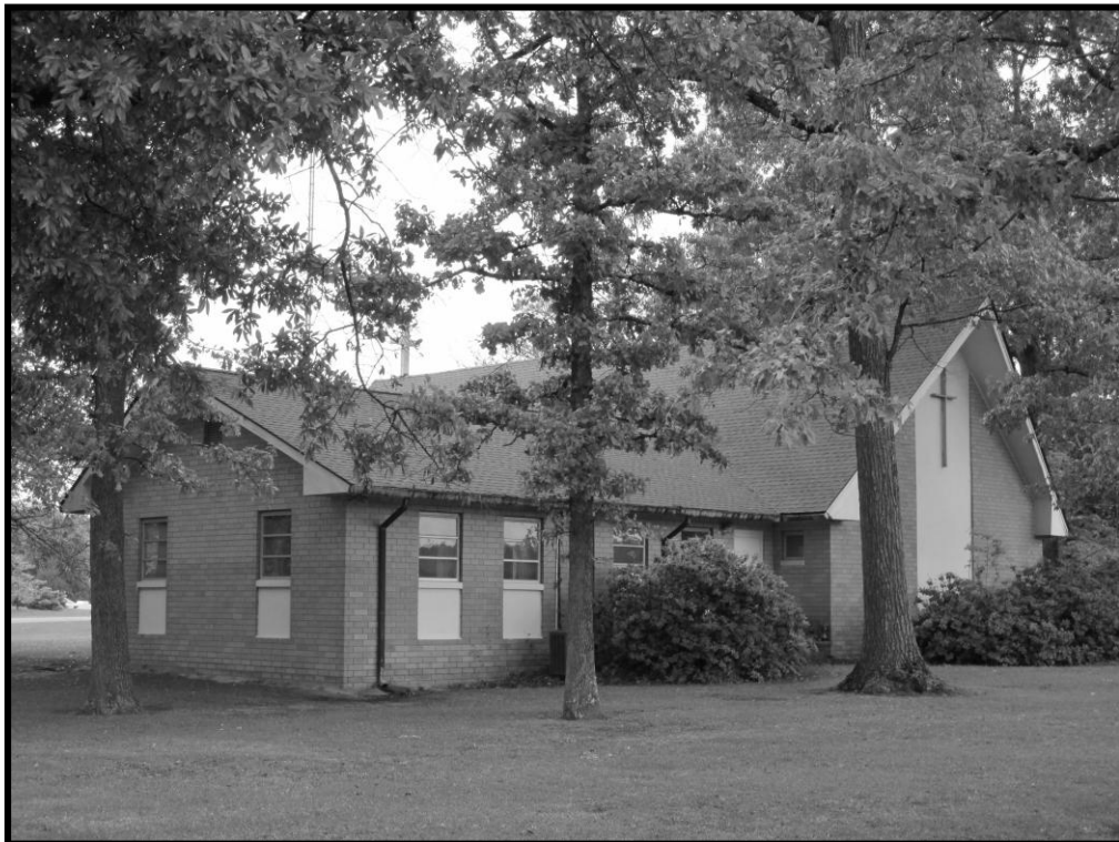
Figure 86. No. 161 Christ the King Catholic Church, View of Northeast Elevation, Looking West.
