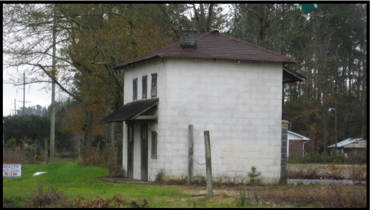
No. 131 (CB155) Concrete Block House
