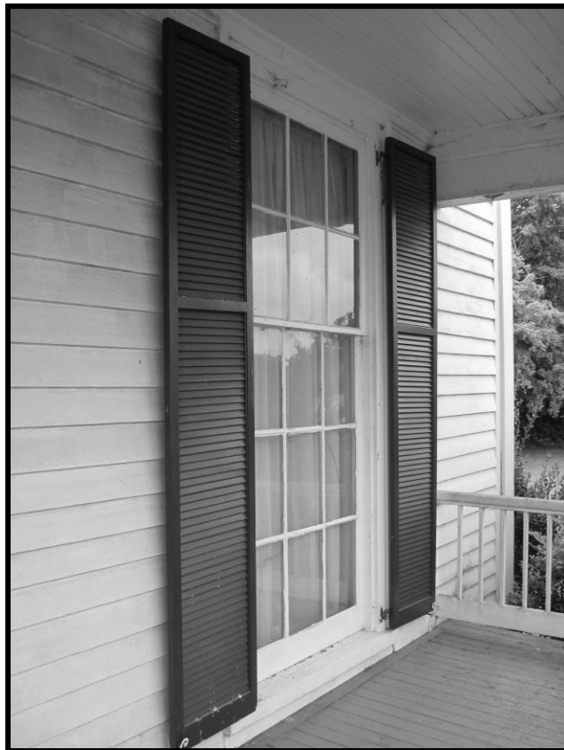
Figure 29. No. 71 Spring Hill, Detail of Sash Window on Northeast Elevation.
