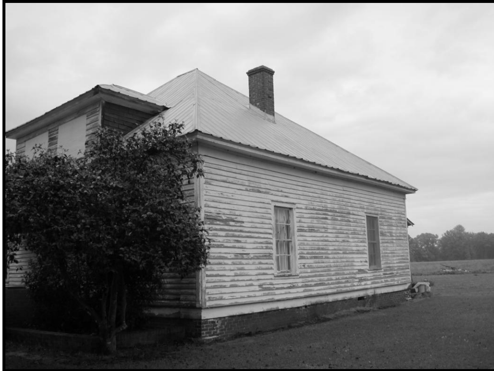
Figure 17. No. 56 Cromartie House, View of Southeast Elevation, Looking North.
