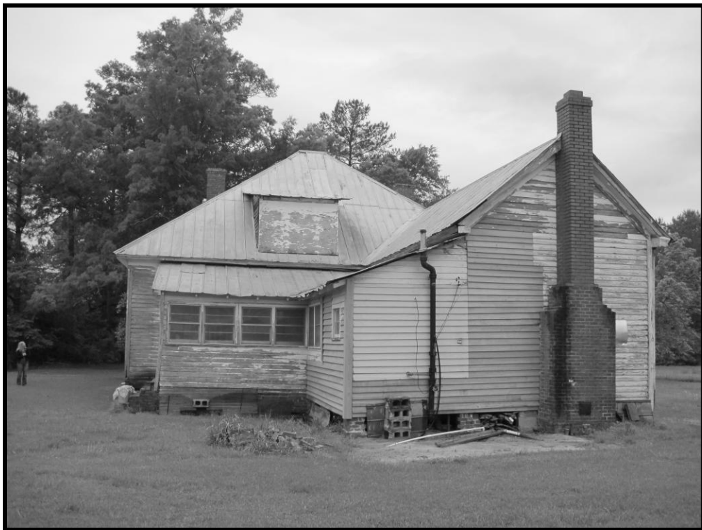
Figure 20. No. 56 Cromartie House, View of Northeast Elevations, Looking West.
