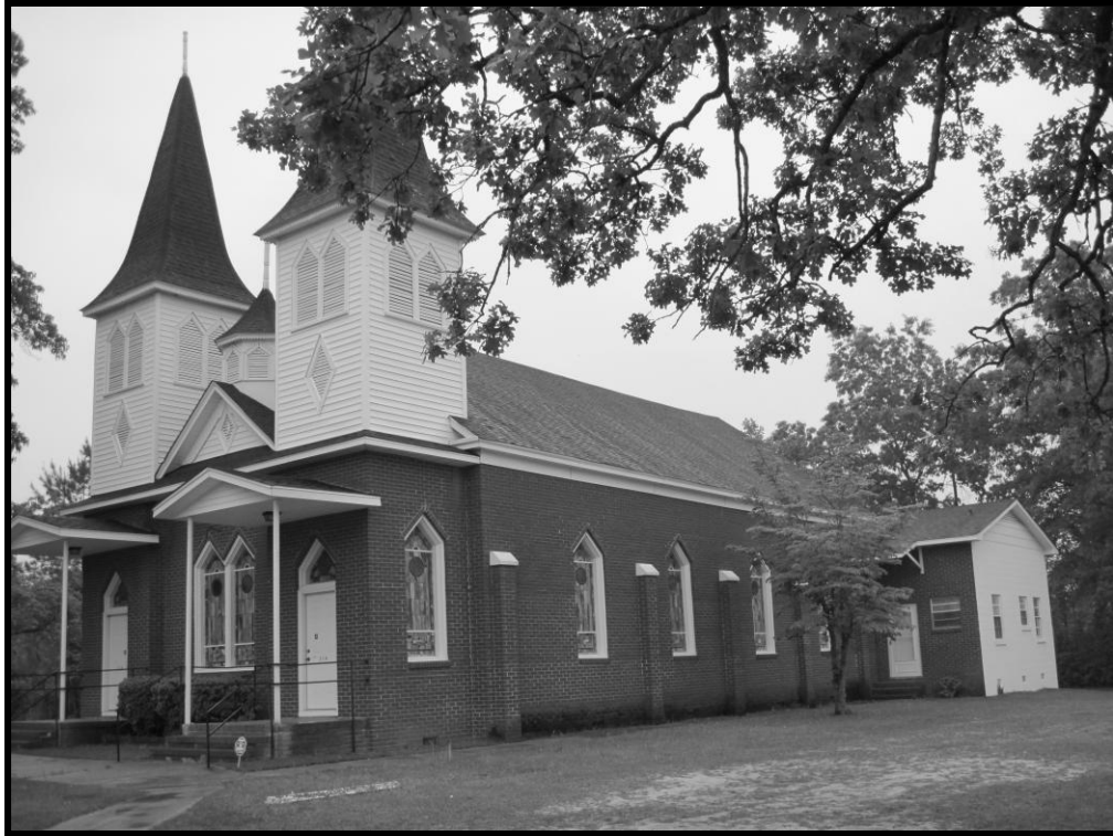
Figure 45. No. 76 Carvers Creek AME Zion Church and Cemetery, View of West and South Elevations of Church, Looking Northeast.
