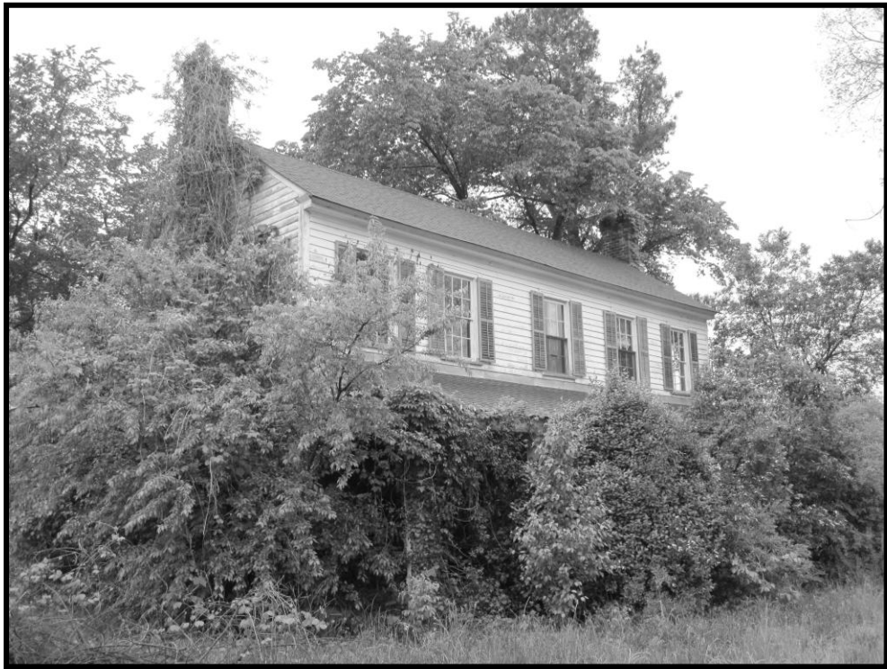
Figure 65. No. 126 Love House, House and Setting, Looking West.
