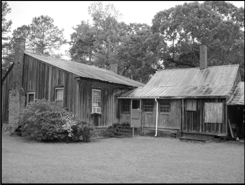
Figure 7. No. 24 McDonald-Russ House, Main House and Kitchen Wing, Looking West.
