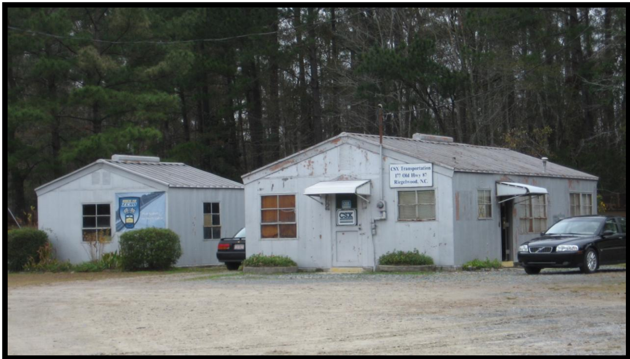
No. 171 (CB192) CSX Transportation
