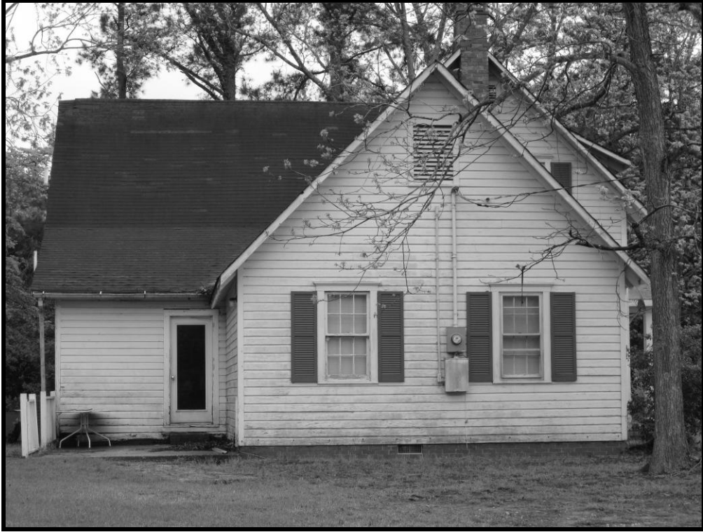
Figure 127. No. 179 Heinzl House, View of Northwest Gable End, Looking Southeast.
