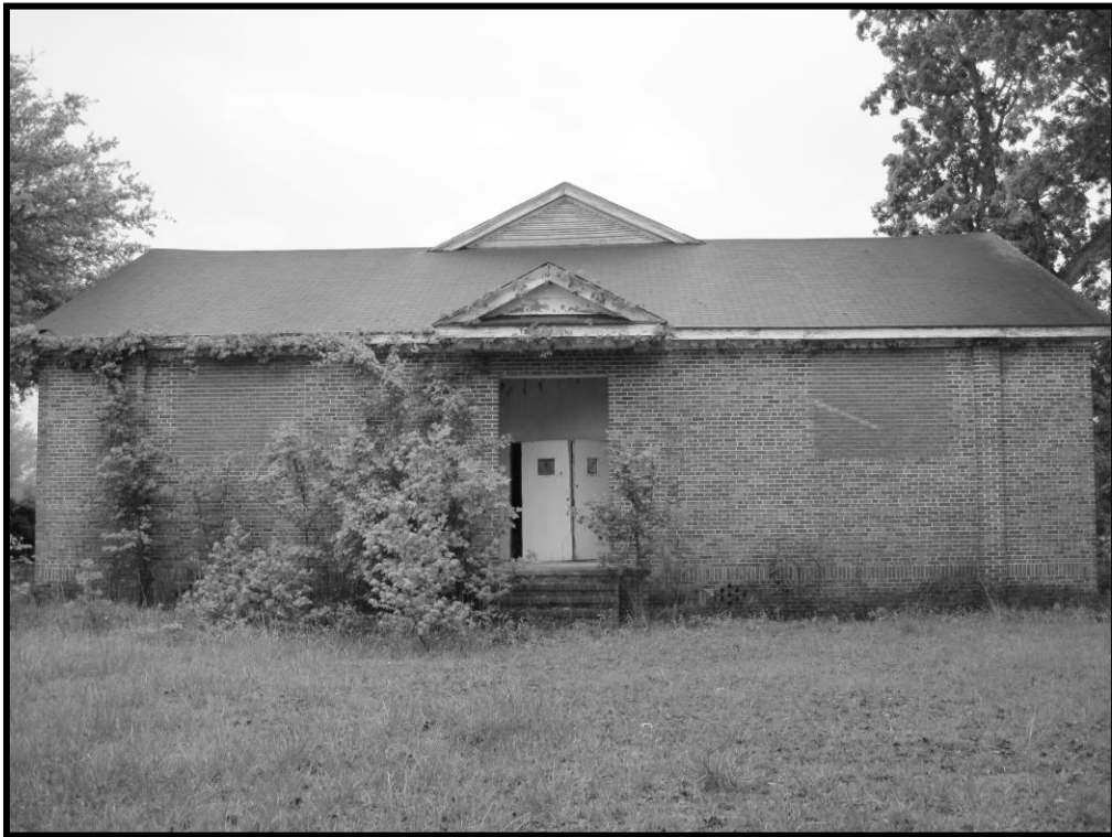
Figure 53. No. 77 Carvers Creek School, View of Northwest Elevation, Looking Southeast.
