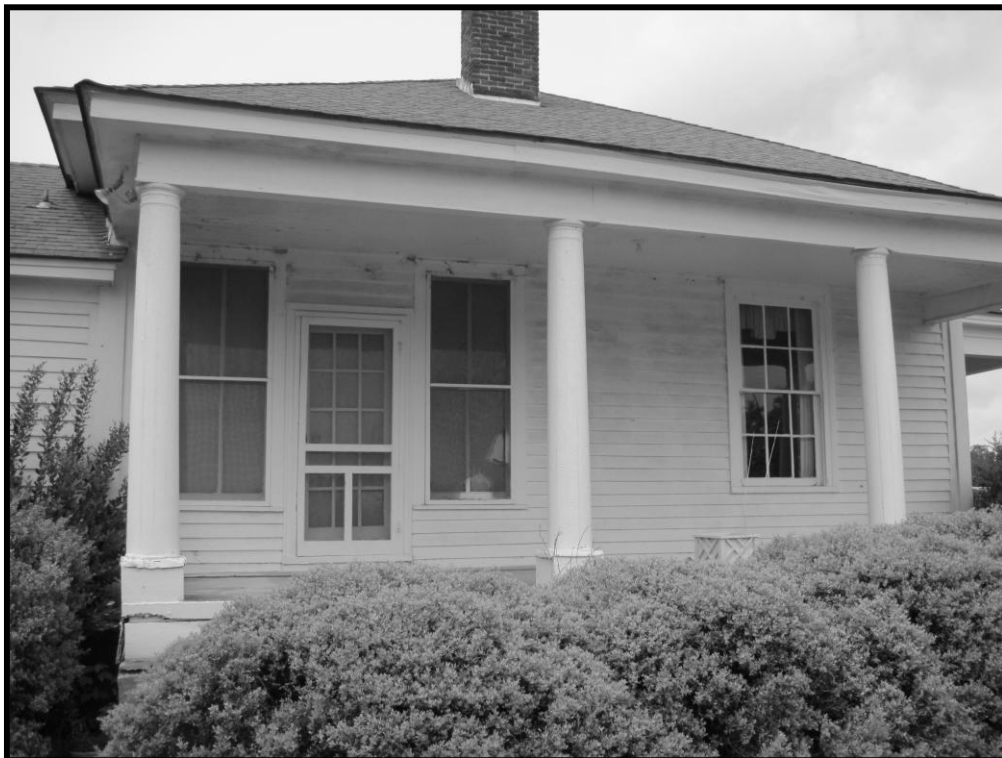
Figure 33. No. 71 Spring Hill, Detail of Porch on Southeast Elevation, Looking North.
