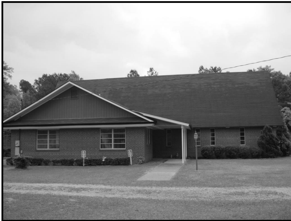
Figure 114. Wesley United Methodist Church, View of Northwest Elevation, Looking Southeast.
