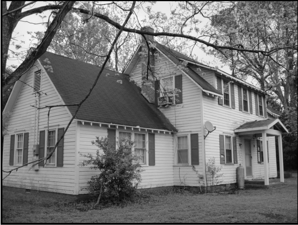
Figure 125. No. 179 Heinzl House, View of the Southwest Elevation, Looking East.
