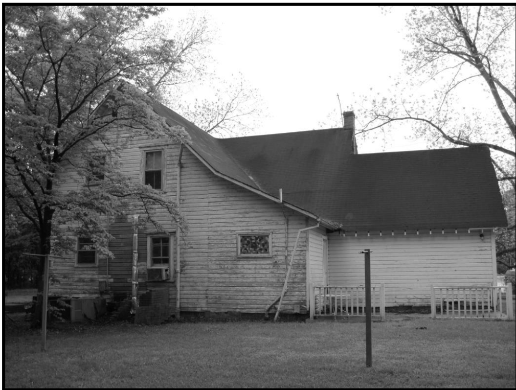
Figure 126. No. 179 Heinzl House, View of the Northeast Elevation, Looking South.
