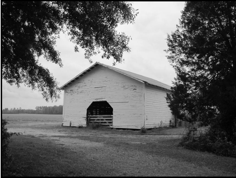
Figure 36. No. 71 Spring Hill, View of Barn, Looking South.
