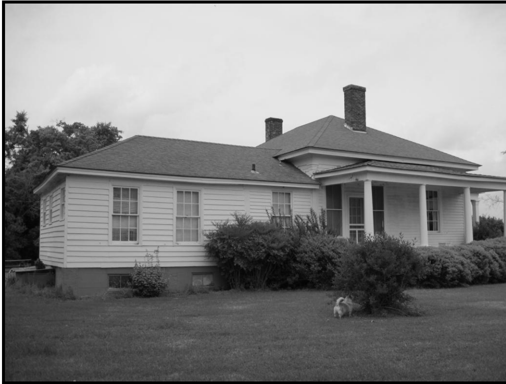
Figure 32. No. 71 Spring Hill, View of Southeast Elevation, Looking North.
