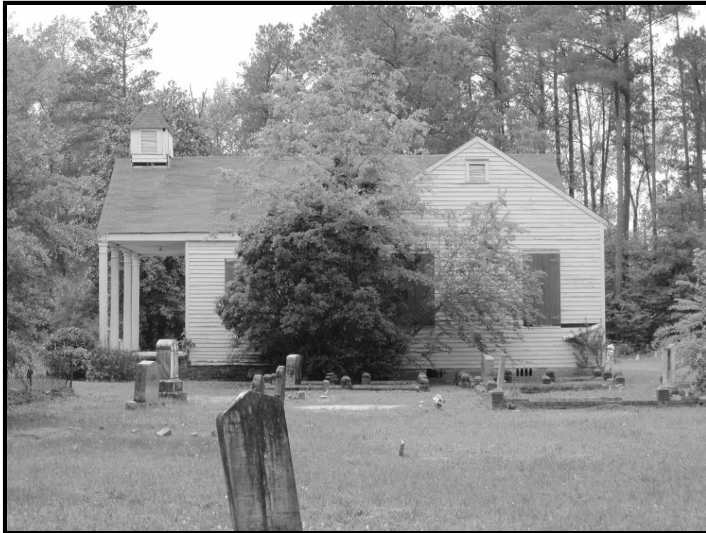
Figure 77. No. 135 Former Weyman Methodist Church, Cemetery and Church, Looking Northwest.
