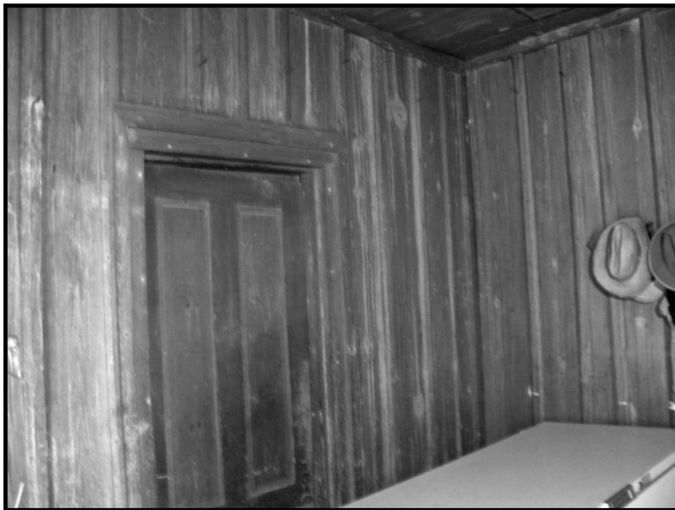
Figure 10. No. 24 McDonald-Russ House, Detail of Board-and-Batten Siding in Original Breezeway of Main Block, Looking South.
