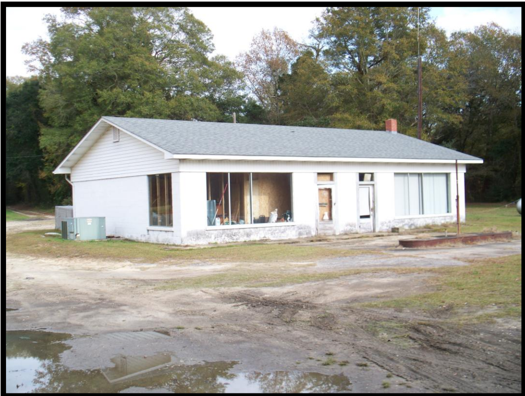
No. 50 (BL314) Store/Gas Station North of NC HWY 87
