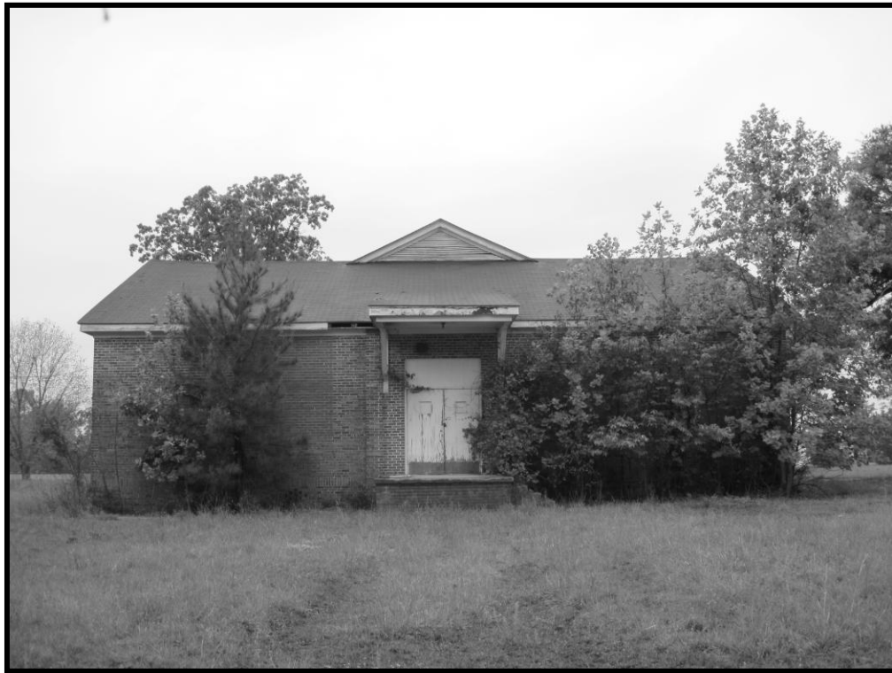
Figure 54. No. 77 Carvers Creek School, View of Southeast Elevation, Looking Northwest.
