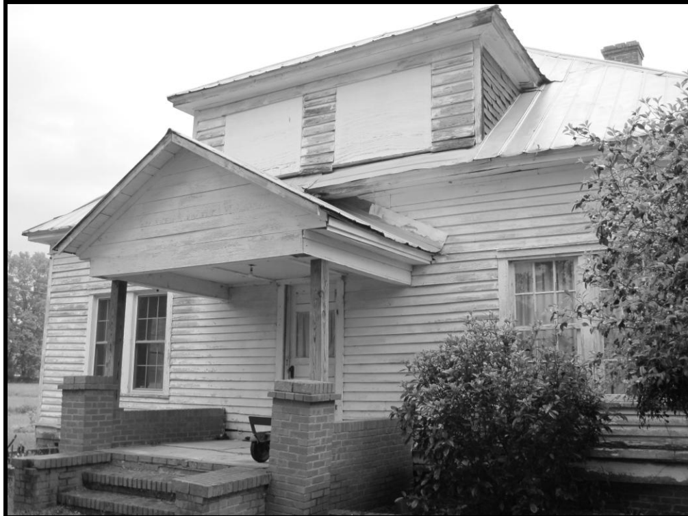
Figure 16. No. 56 Cromartie House, View of Southwest Elevation, Looking North.
