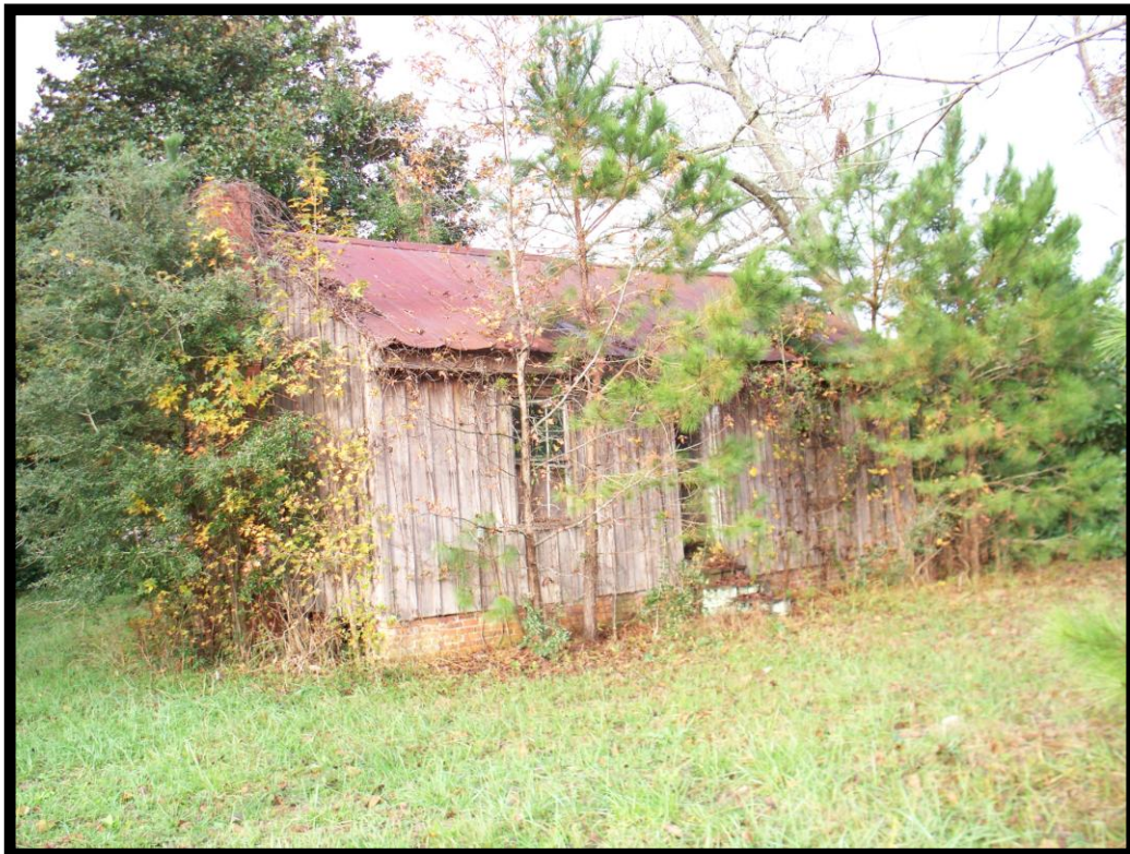
No. 66 (BL328) Three Houses, House A, West Side of NC HWY 87
