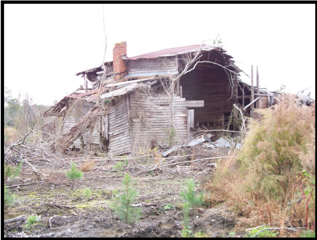
No. 69 (BL331) Old General Store, North Side of SR 1725
