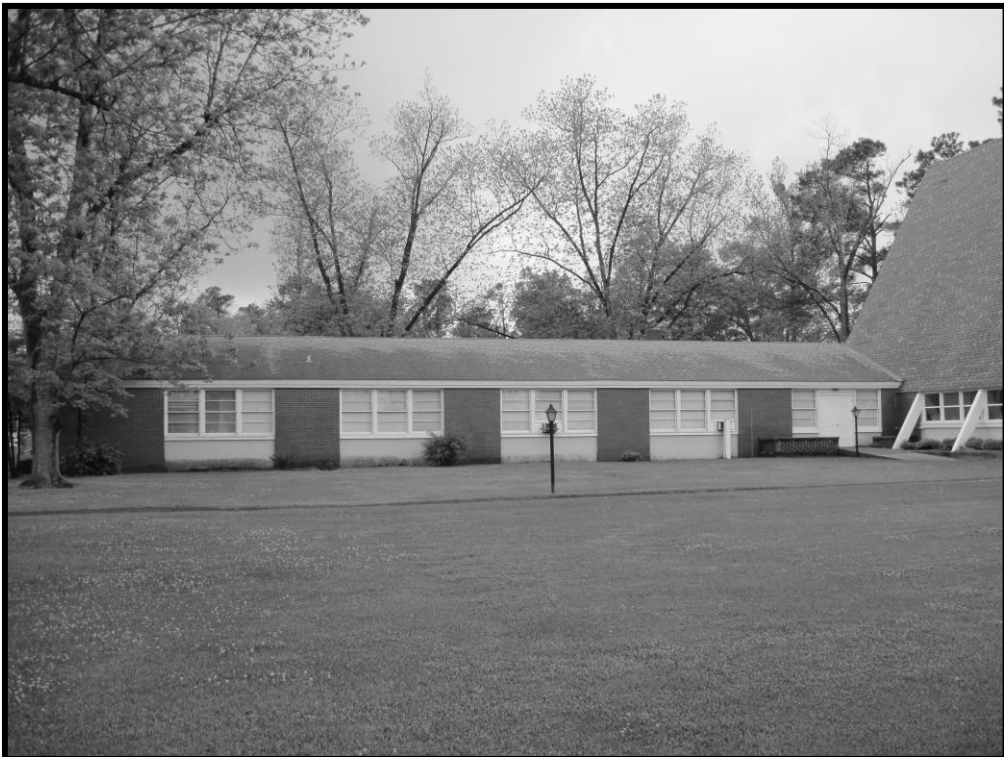
Figure 97. No. 163 Acme Presbyterian Church, View of Sunday School Wing, Looking Southwest.
