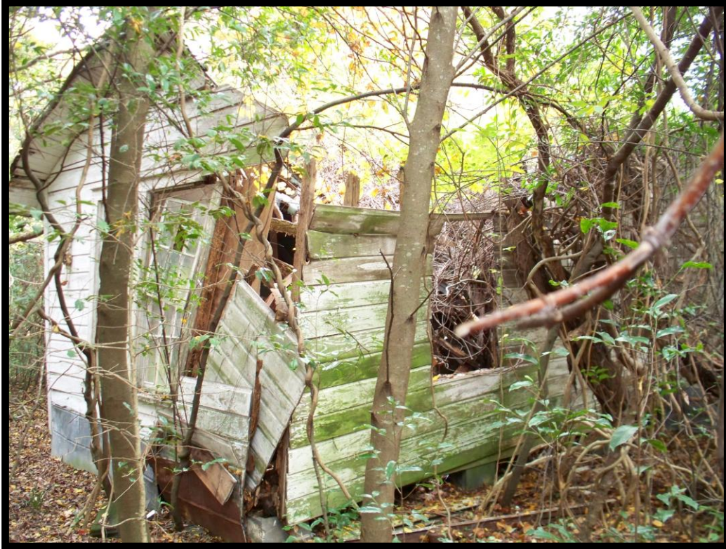
No. 9 (BL275) Collapsed House
