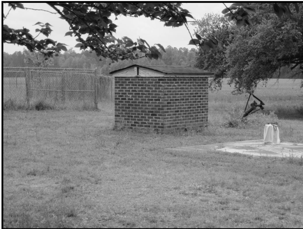
Figure 39. No. 71 Spring Hill, View of Pump House, Looking Southwest.
