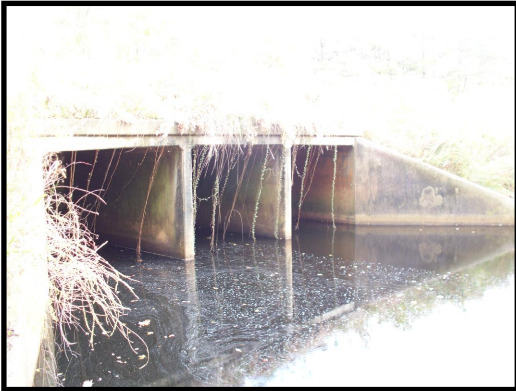
No. 82 (BL341) Culvert, HWY NC 87 over Carvers Creek
