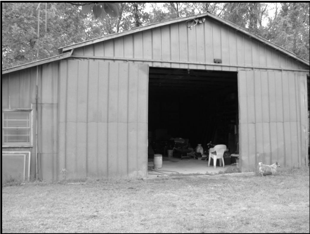
Figure 37. No. 71 Spring Hill, View of Machine Shed, Looking West.
