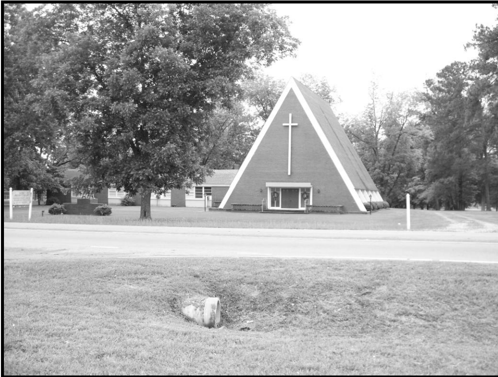
Figure 98. No. 163 Acme Presbyterian Church, Church and Setting, Looking Southwest.
