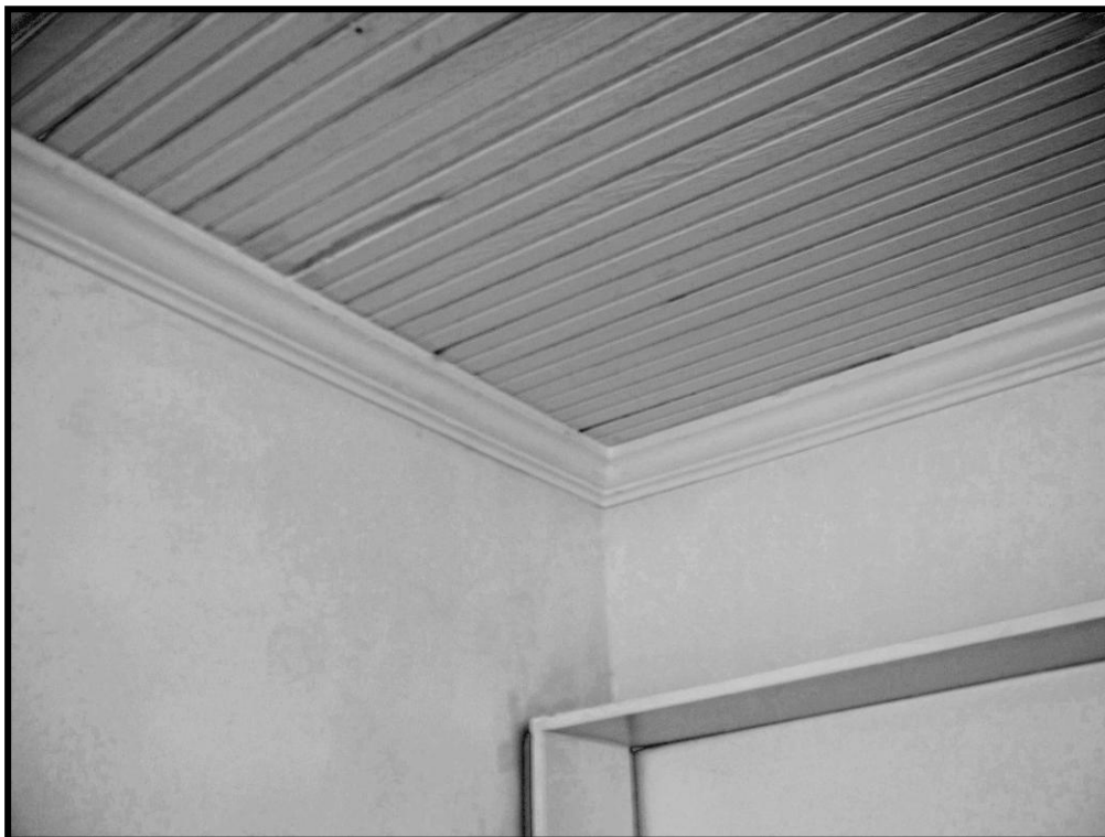
Figure 130. No. 179 Heinzl House, Interior, Detail of Narrow Board Ceiling and Crown Molding.
