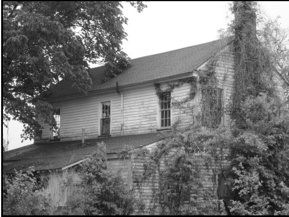
Figure 67. No. 126 Love House, View of Southwest Elevation, Looking North.
