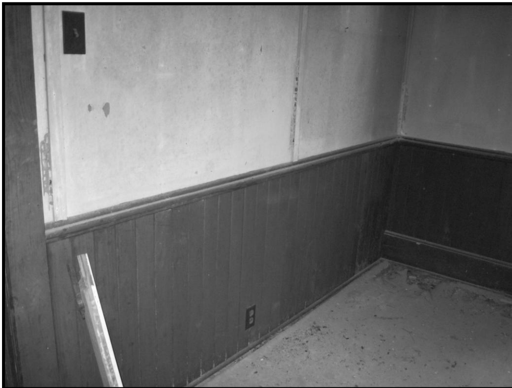
Figure 82. No. 135 Former Weyman Methodist Church, Interior, Detail of Beaded Board Wainscot in Sunday School Rooms.
